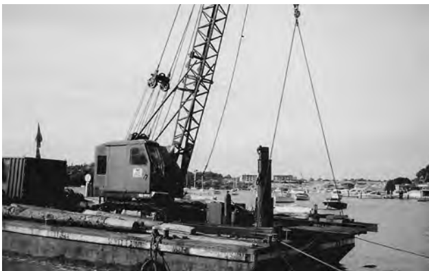
The new pontoon is lifted into place by a floating crane.
