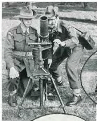
Left: Correcting aim on 3" mortar.
